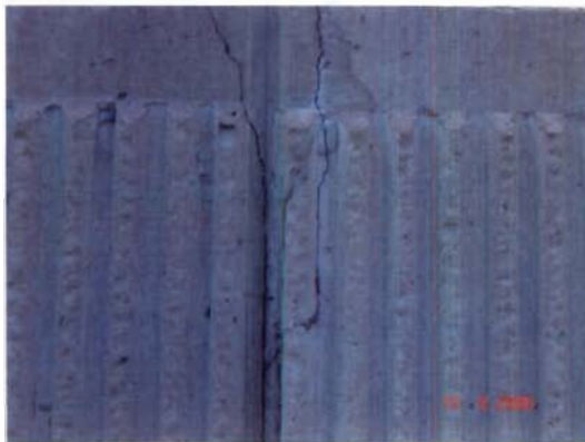
Photo 18. Hairline joint cracks east of Grant and south of river riverside.
