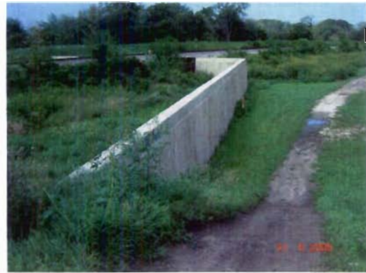
Photo 4. Floodwall west of Burr Street at NS railroad.
