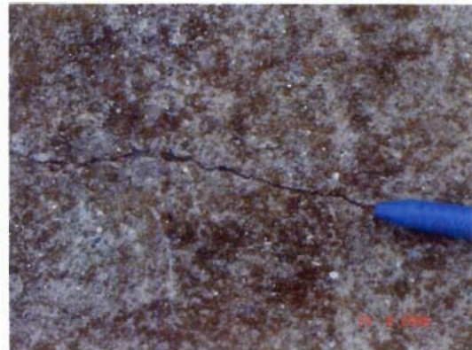
Photo 15. Hairline crack at utility crossing west of Broadway.
