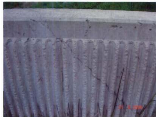
Photo 16. Hairline crack on landward side at Georgia Street south of river.
