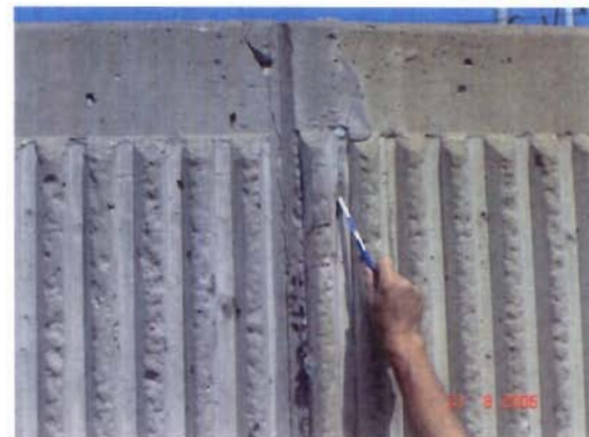
Photo 22. Hairline joint cracks east of Grant and south of river landside.
