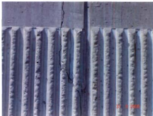
Photo 19. Hairline joint cracks east of Grant and south of river riverside.
