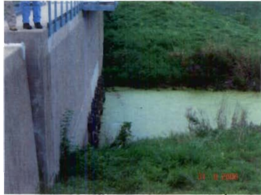
Photo 25. Inaccessibility along 35 th Street between Chase and Grant.
