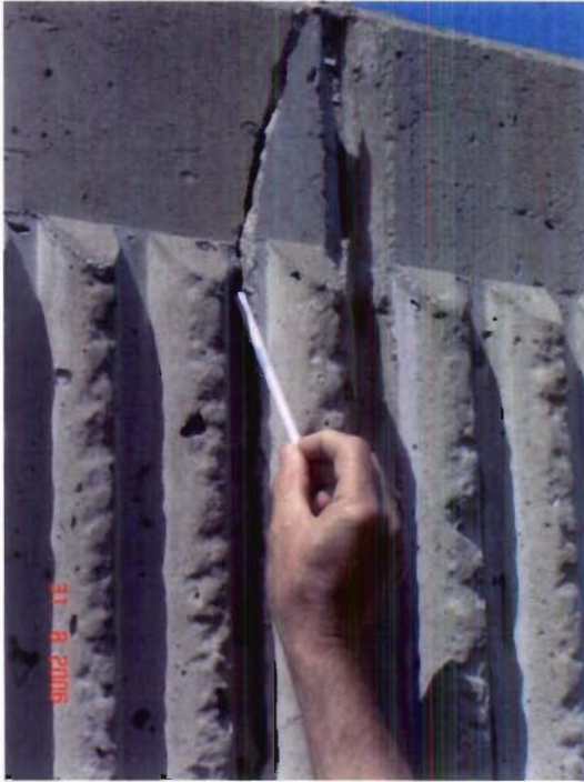
Photo 23. Cracking west of Grant and south of river landside.
