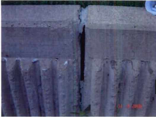
Photo 17. Missing caulk south of river and east of Broadway.
