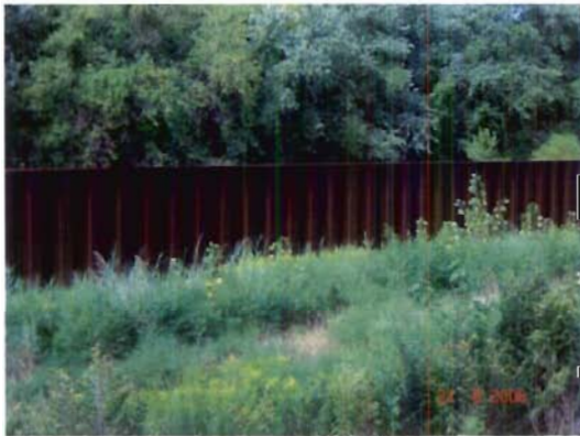
Photo 2. Landward side of wall east of Colfax Ave and north of river.
