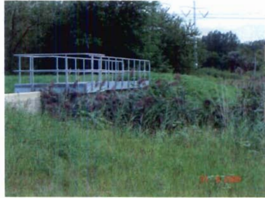
Photo 14. High grass obstruction east of Grant and north of river.
