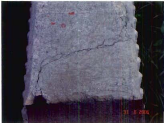
Photo 7. Hairline cracking at concrete to steel transition west of Burr south of RR.
