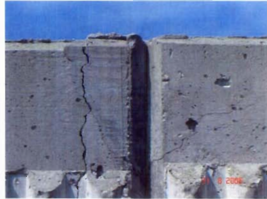
Photo 20. Hairline joint cracks east of Grant and south of river landside.
