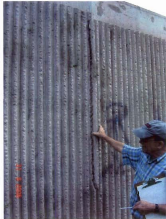
Photo 5. Cracking of the fractured fin finish (landside).
