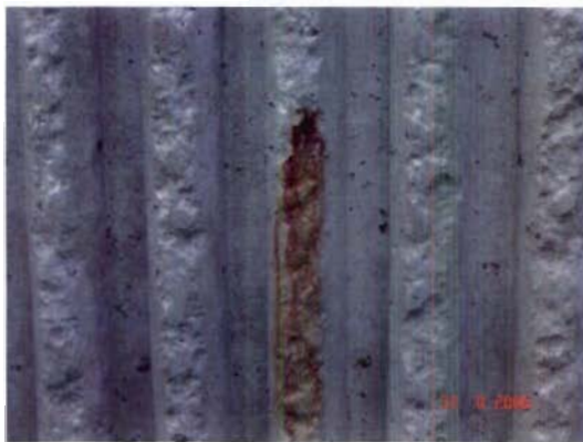
Photo 8. Typical rust staining on concrete.
