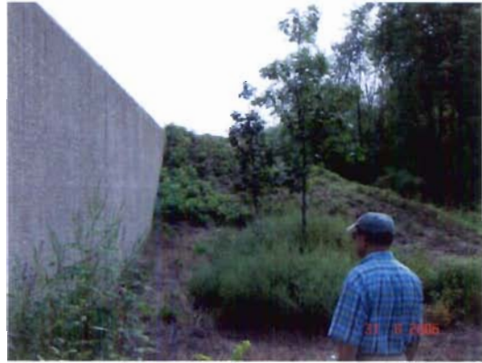
Photo 9. Concrete T-wall east of Burr Street.
