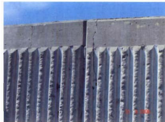
Photo 21. Hairline joint cracks east of Grant and south of river landside.
