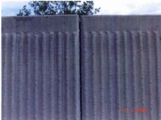
Photo 12. Opening at control joint west of Grant Street and north of river.
